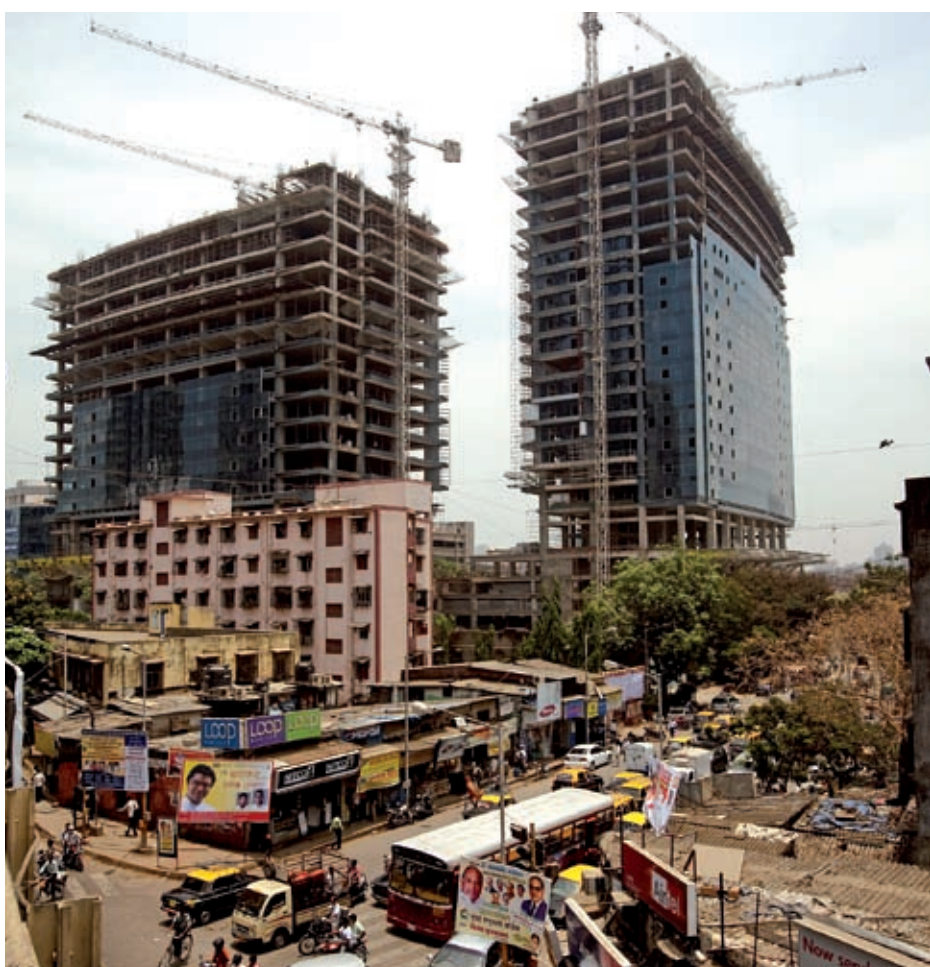
New commercial buildings being constructed in Mumbai, India. While the significance of China is widely discussed today, an increasing number will be discussing India in future.
